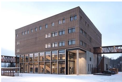
Project name: NTNU Gjøvik University Architect name: Reiulf Ramstad Arkitekter Category: Higher Education and Research Country: Gjøvik, Norway
