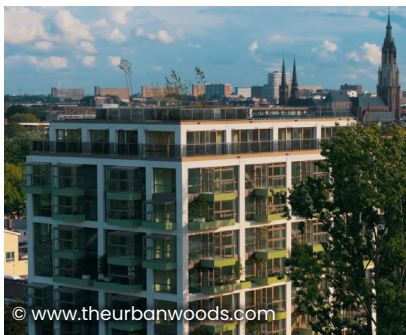
The Urban Woods is a 10-storey, low-carbon, residential development constructed entirely of CLT panels. Demolition wood and discarded pallets, all sourced locally in the Netherlands, were used to manufacture the CLT.
