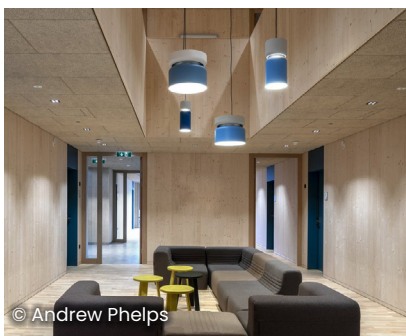
The Wood Technology Association boarding school in Kuchl, Austria, used over 1,000 m 3 of CLT, supplied by Mayr-Melnhof in its construction.
