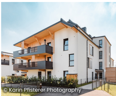
This development by Siges Massivholzbau, comprises 80 apartments. 3,000 m 3 of wood, partly sourced from local PEFC-certified forests, was used in its construction, making it one of the largest multi-story wooden residential buildings in Salzburg, Austria.
